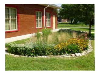
Rain Gardens: Stormwater can be diverted into shallow landscaped depressed areas or rain gardens where vegetation cleans the water and allows it to soak into the ground. Rain gardens come in all shapes and sizes and can be designed to disconnect rooftops, driveways, patios, and parking areas.
