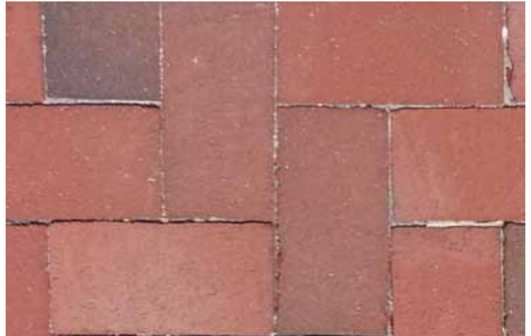
Above: Permeable pavers blend in with existing brick. A thick grout/gravel line is the only discernible difference.
