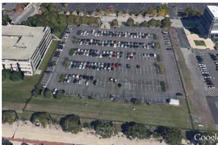
Above: The Federal St. surface parking lot, in its current layout. Short and long-term options include taking advantage of the lot's size and wide yard fronting the street.
