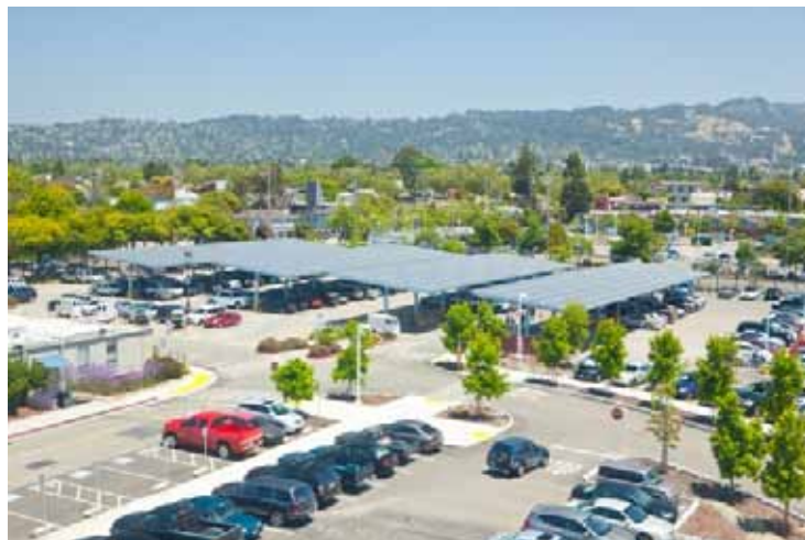
Above: This parking lot in Berkley, CA provides solar panels, permeable pavements and landscaping.
