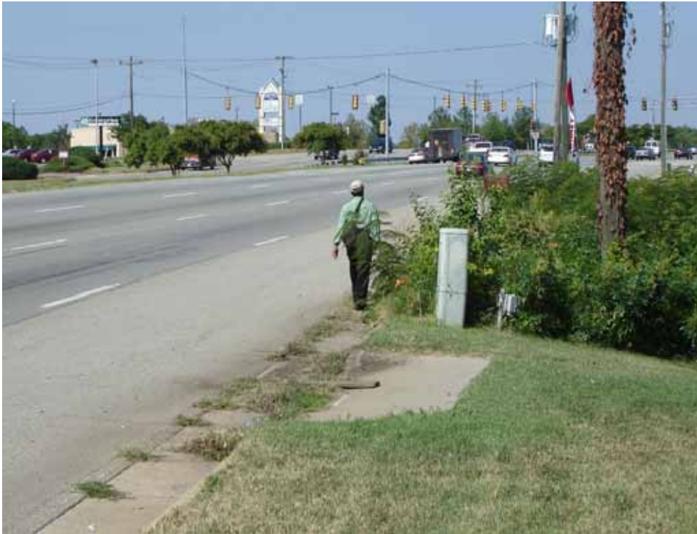
Above: Incomplete sidewalks and crosswalks force pedestrians to walk in travel lanes.
