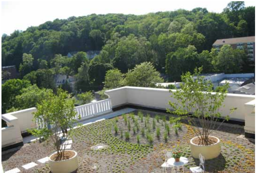
Above: A green roof installation on the Geraldine R. Dodge Foundation headquarters in Morristown, NJ. In addition to its stormwater benefits, the native plant rooftop provides bird habitat in a downtown setting.
