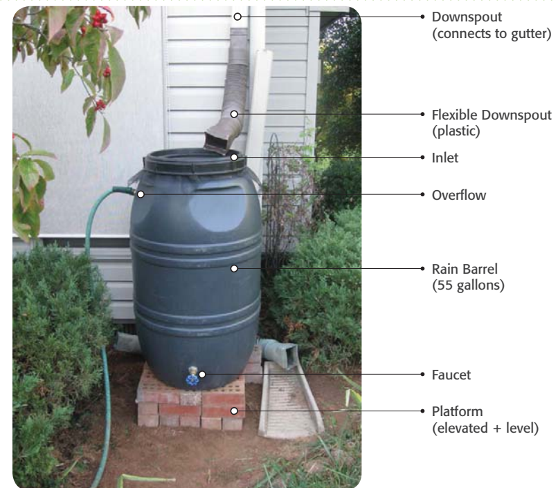
Example of a residential rainwater harvesting system
